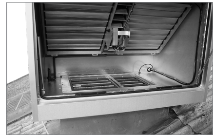
Fig. 43: Extract air filter
